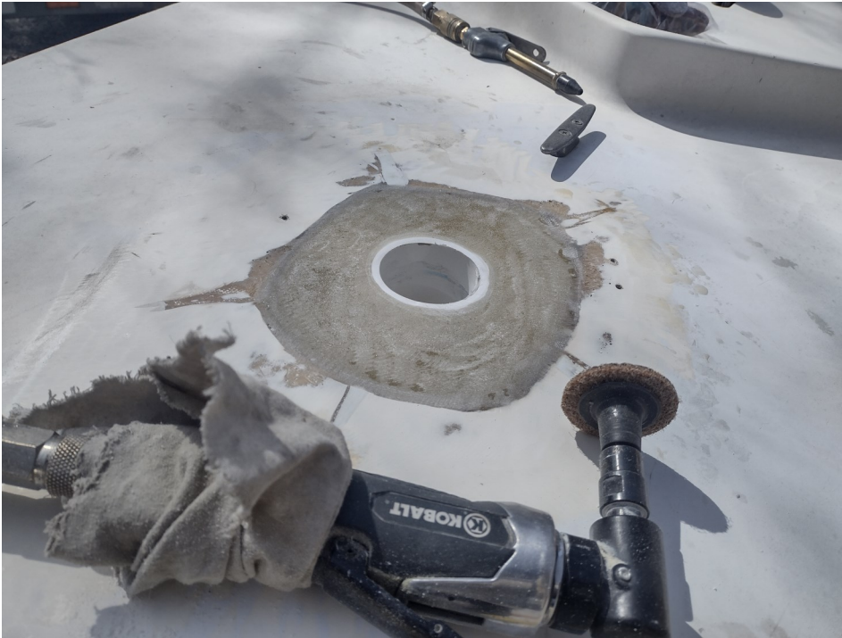
08 Smoothed for fiberglass tape
