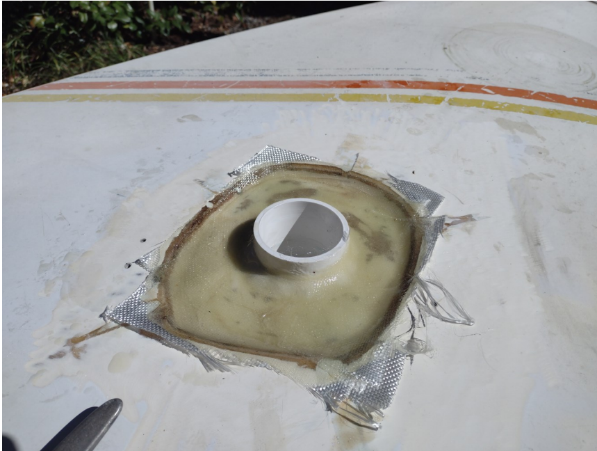
06 Approximately 12 plies of fiberglass tape
