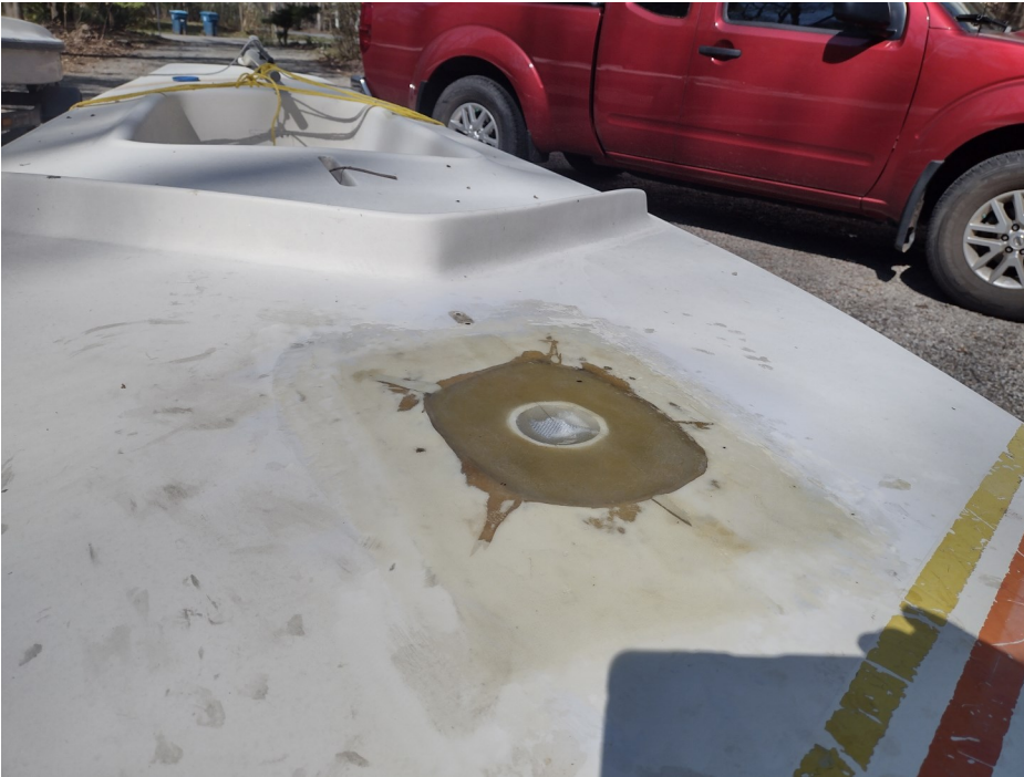
10 Sanded—fill coat applied
