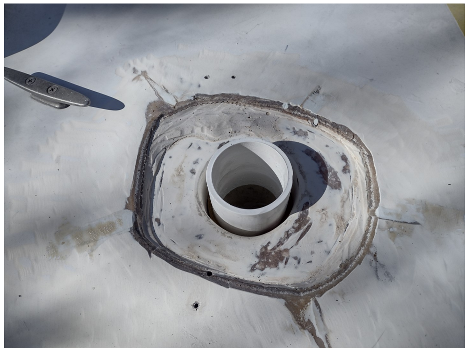
03 Smoothed, 2 inch PVC coupling inserted
