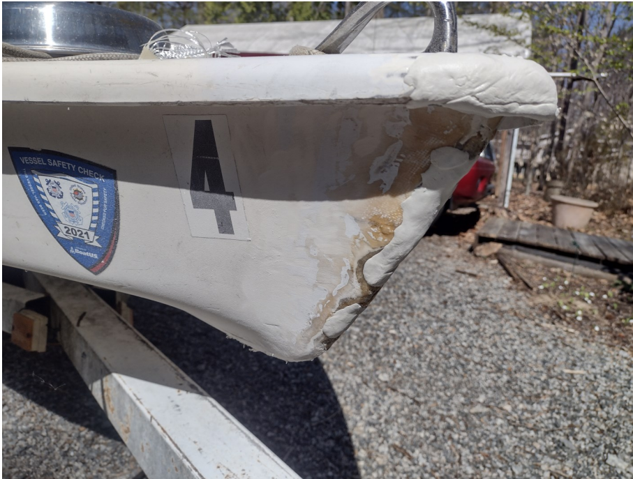
02 Epoxy putty to support fiberglass
